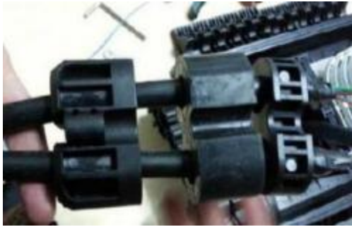
4.4 After the cable passing through the ports into the box, tighten the hose clamps, fixing cable.
